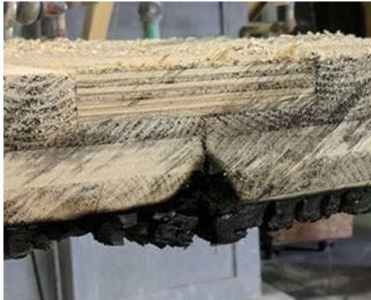
Figure C3-1 Example of char penetration at abutting edges of CLT floor panels likely caused by gap formation due to bending deformation (photo courtesy of Katerra).
