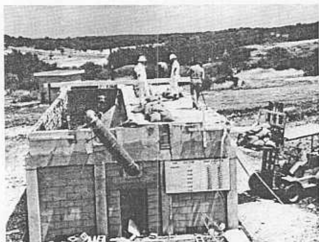
Figure 8. Exterior view of the test structure after the test showing workmen unloading the wood supported panel prior to removal for inspection and measurement of the wood beam.
