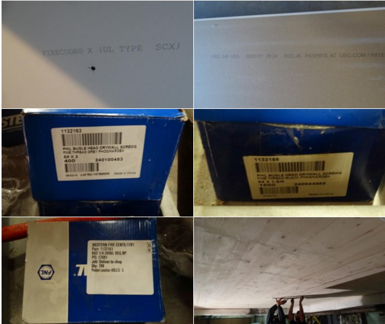
Figure A 2. Construction showing (a) Test 1 joint, (b) firestop, (c) construction adhesive, (d) spline screws, (e-f) gypsum, (f) 3” screws, (g) 1<sup>5</sup>/<sub>8</sub>” screws, (h) 2<sup>1</sup>/<sub>4</sub>” screws, and (i) underside CLT.
