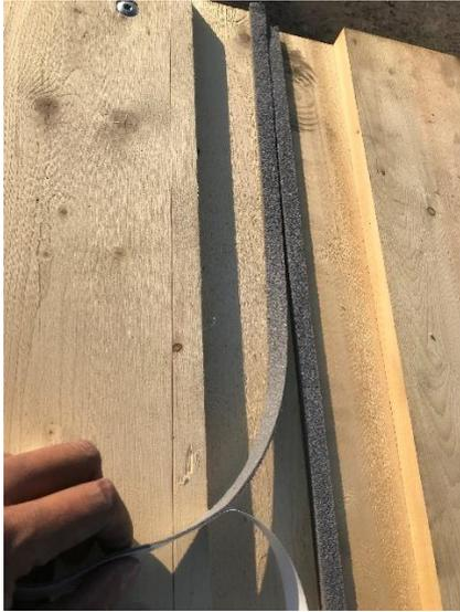
33 - Test 2. Installing expanding foam tape on the ceiling joint.
