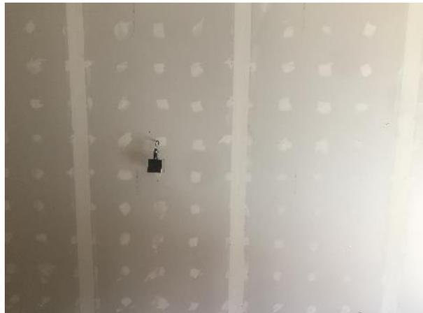
8 - Test 1. Back wall after gypsum board installation
