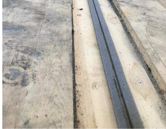
Figure 91: Photo after removal of spline board. Sealing method: 2x expanding tape under spline board at CLT interface (Test 2)
