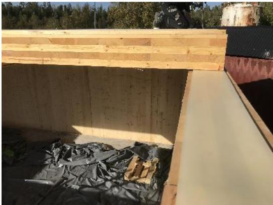
31 - Test 2. Resilient profile between wall and ceiling.
