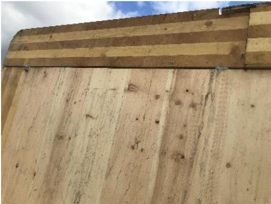
35 - Test 2. Wall-ceiling joint from outside before tape installation.
