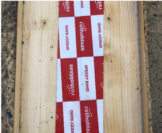
Figure 92: Photo after removal of spline board. Sealing method: construction tape under spline boards at CLT interface (Test 4)
