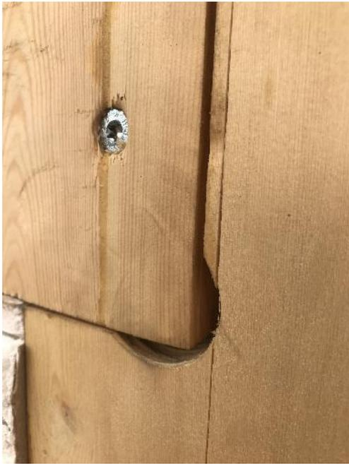
9 - Test 1. Lap joint above corners of openings, without sealant in Test 1
