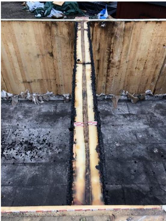
125 - Beam post fire after ceiling removal. Resilient profiles still in place.
