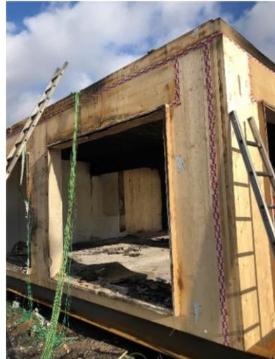
Figure 100: Test 4 - Left façade after removal of gypsum boards.
