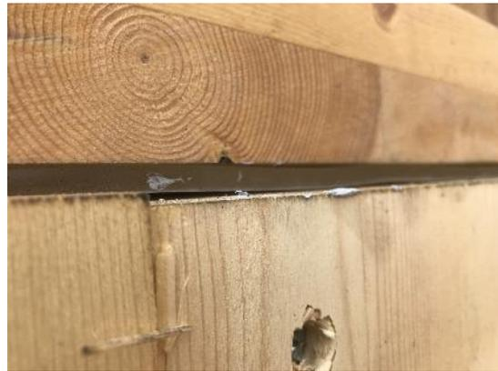
36 - Test 2. Wall-ceiling joint from outside before tape installation.
