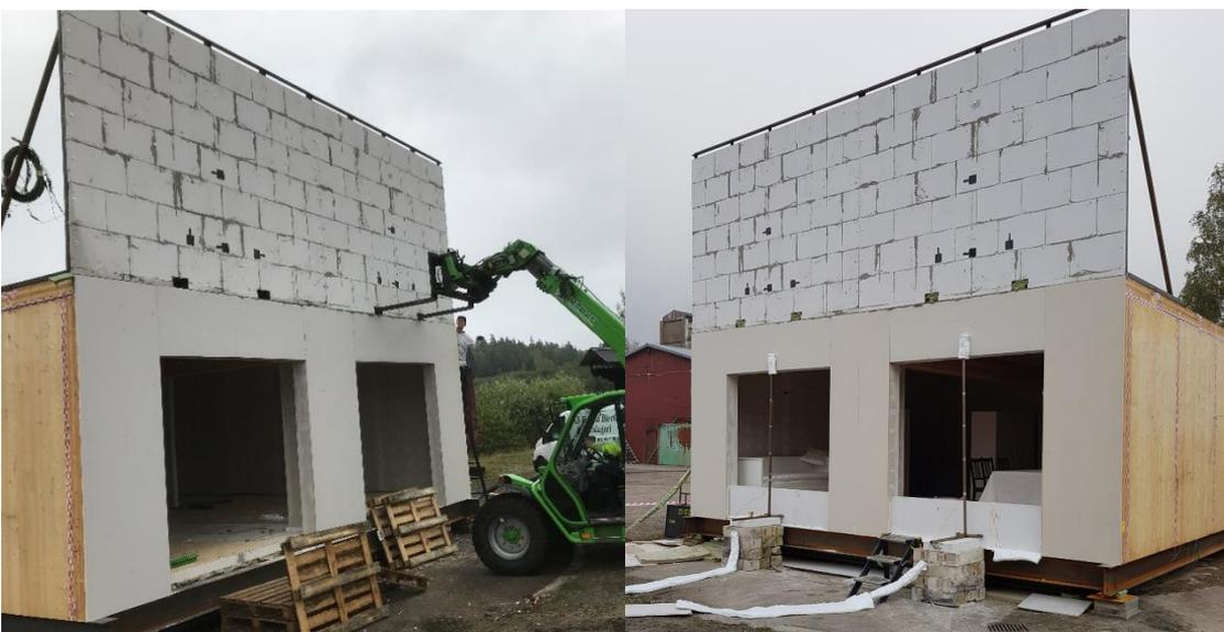
Figure 16: Placement of a façade segment on the construction (left). Facades in place prior to test 1.
