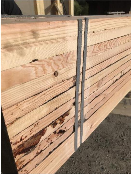
29 - Test 2. Expanding tape to seal where the beam penetrates the back wall.
