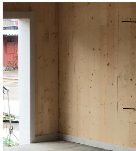
67 - Test 3. Exposed CLT wall in a corner.
