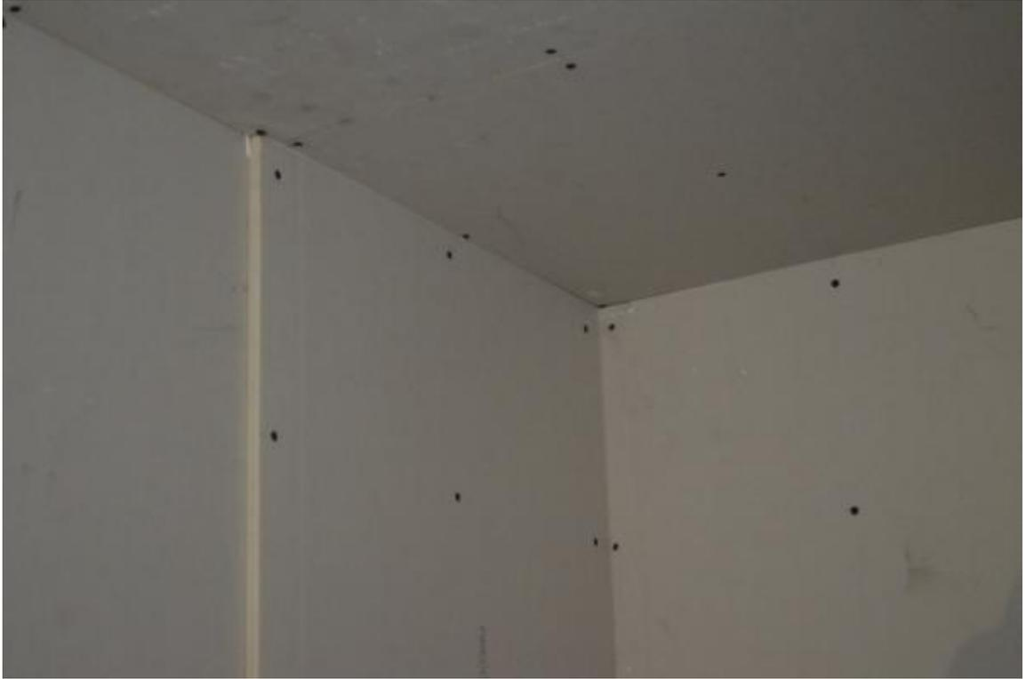
**Figure B-7. Face Layer of Gypsum Board on Walls.**
