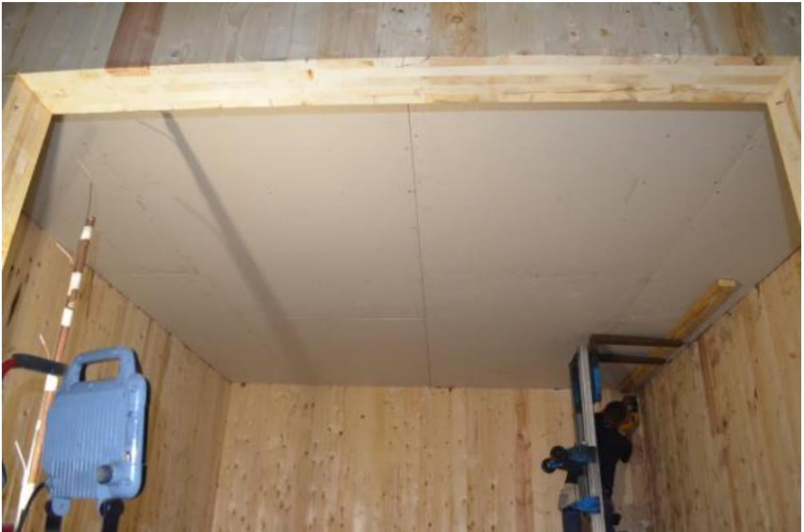
**Figure B-4. Base Layer of Gypsum Board on Ceiling.**
