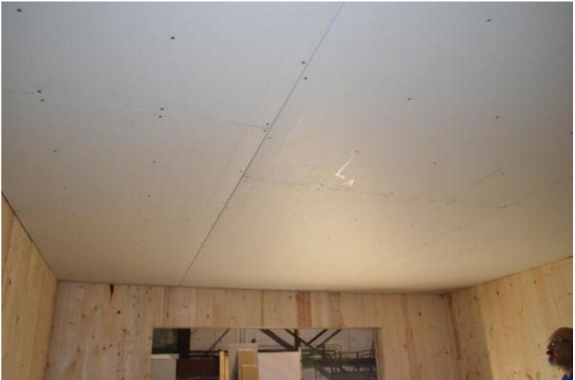
**Figure D-6. Base Layer of Gypsum Board on Ceiling.**
