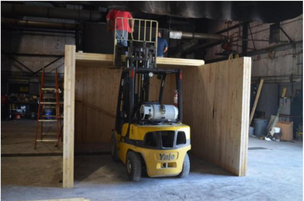
**Figure D-2. CLT Ceiling under Construction.**
