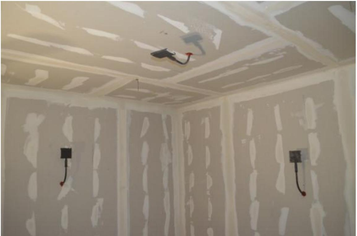
**Figure D-10. Gypsum Board Joints Taped and Floated.**
