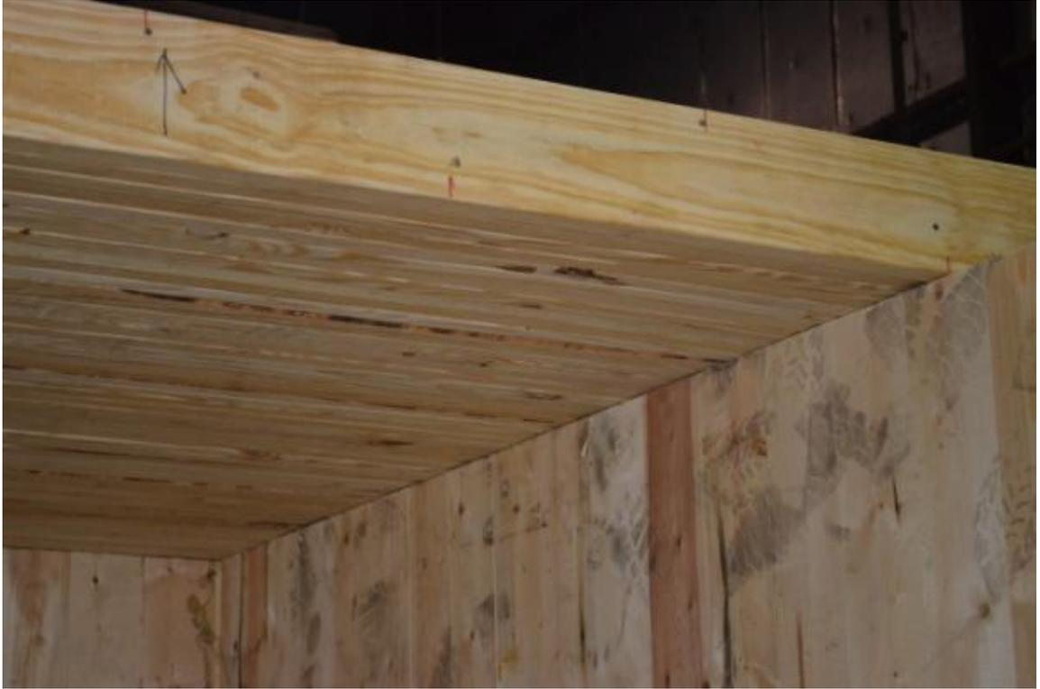
**Figure B-3. NLT Ceiling under Construction.**
