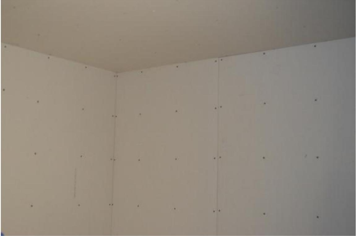
**Figure D-7. Base Layer of Gypsum Board on Walls.**
