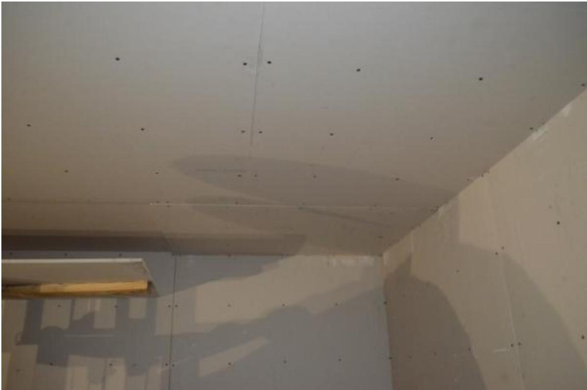
**Figure D-8. Face Layer of Gypsum Board on Ceiling.**
