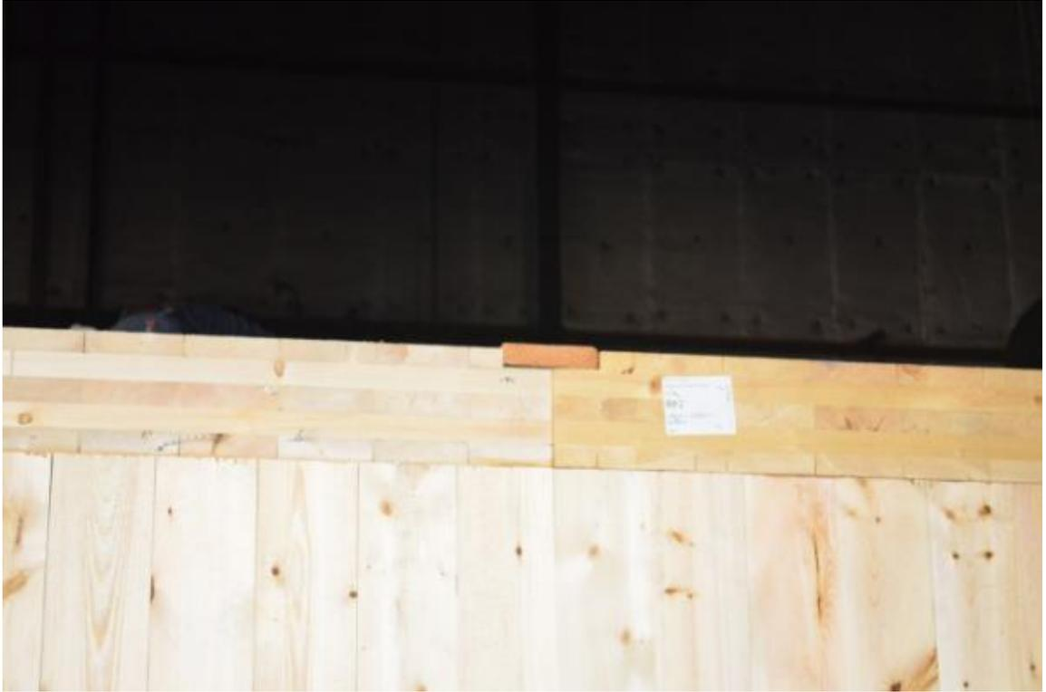
**Figure D-3. Spline Covering Joint between CLT Ceiling Panels.**
