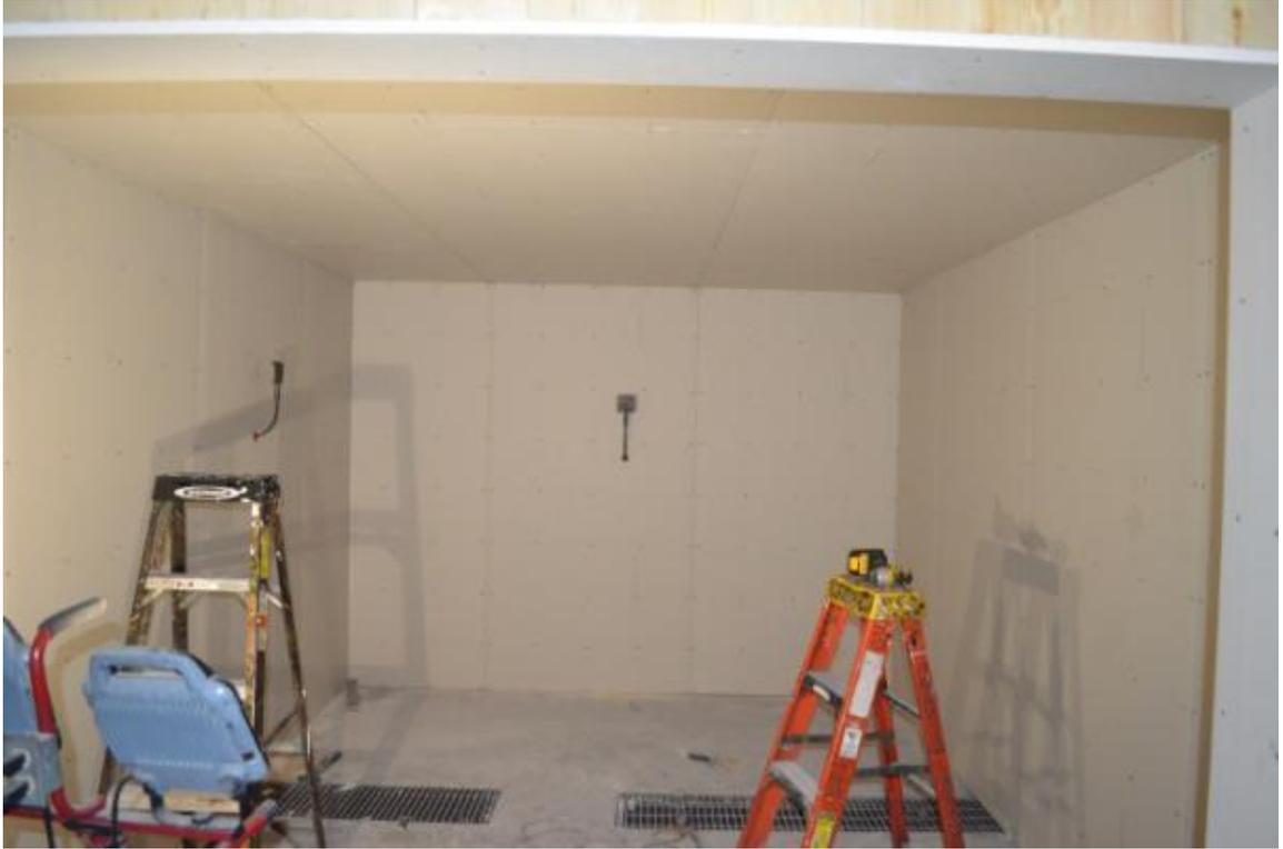
**Figure D-9. Room with Face Layer of Gypsum Board on Walls.**
