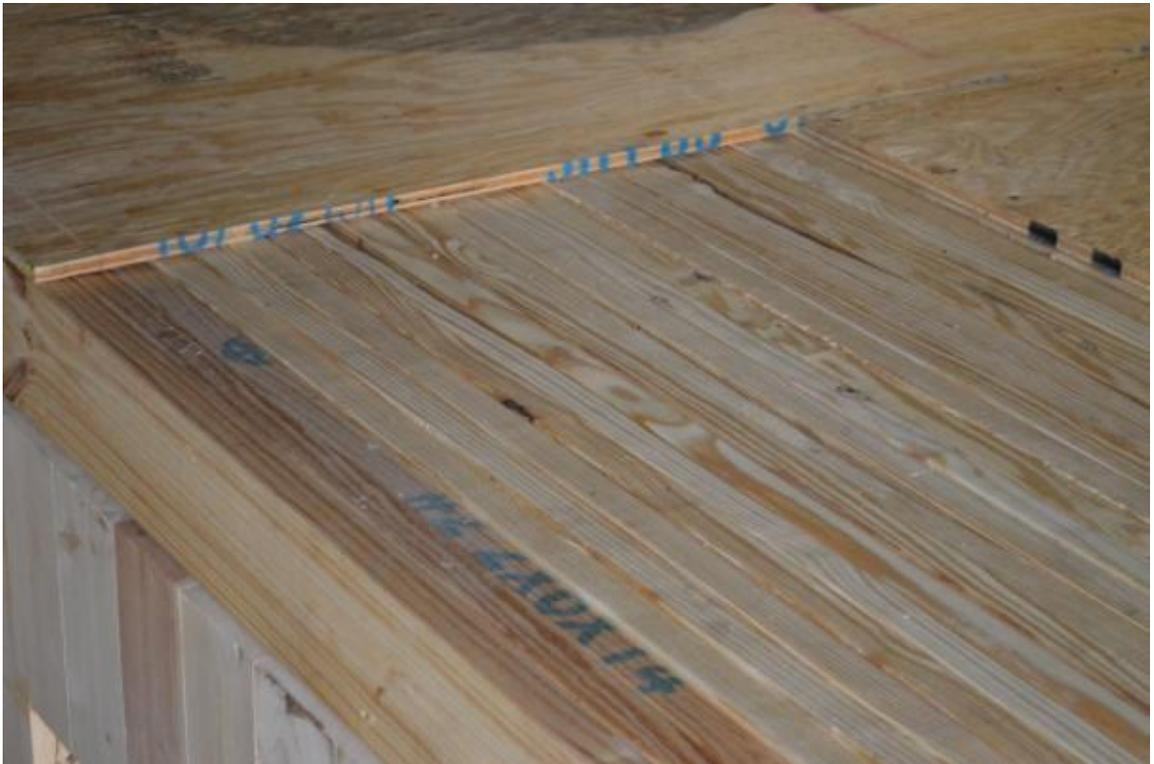
**Figure B-10. Plywood on NLT Ceiling.**
