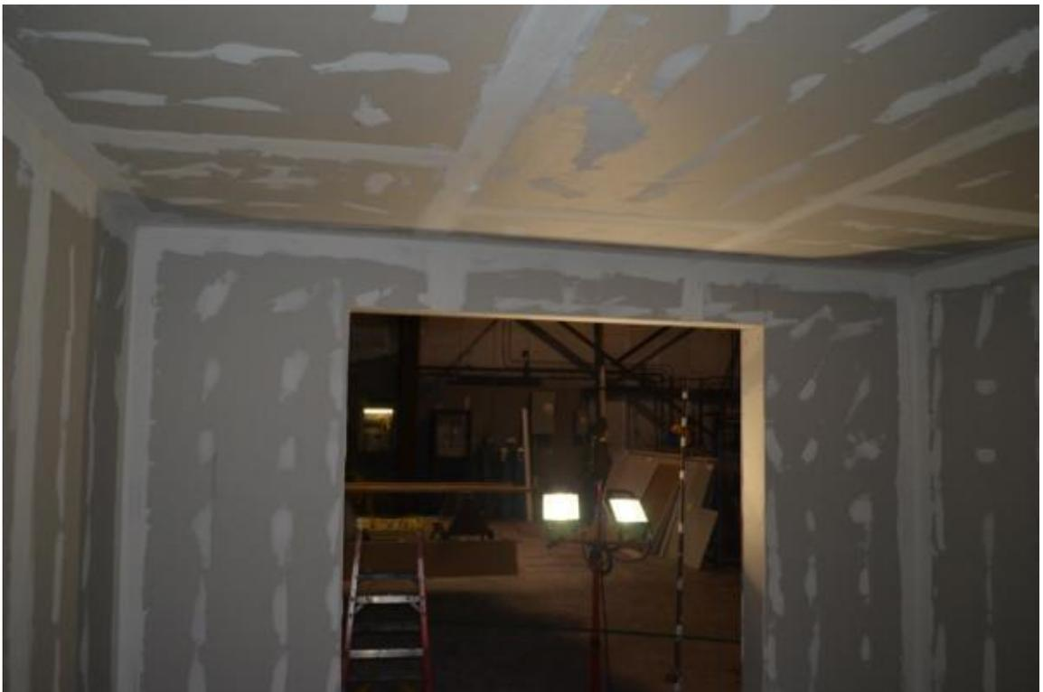
**Figure B-8. Gypsum Board Joints Taped and Floated.**
