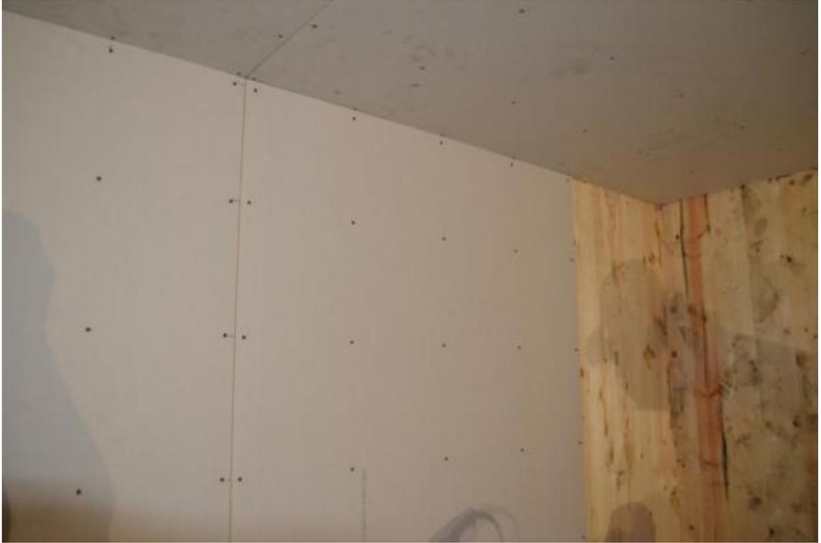
**Figure B-5. Base Layer of Gypsum Board on Walls.**
