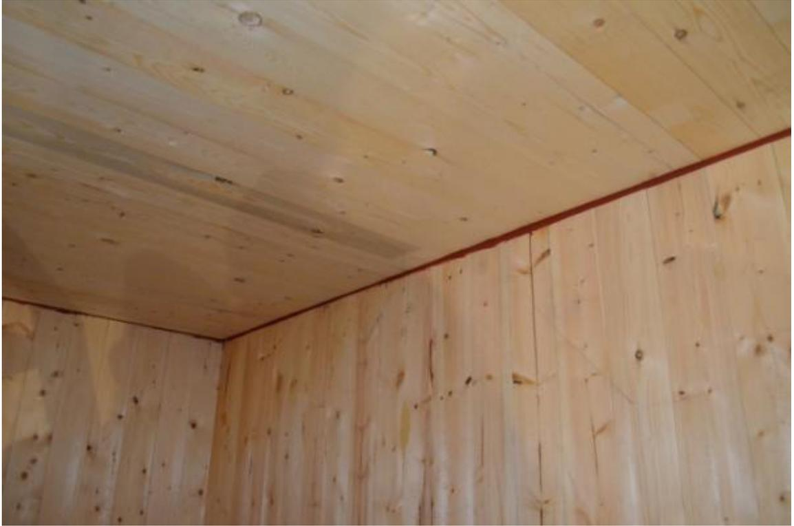
**Figure D-5. Fire Sealant around Room Perimeter at Wall-Ceiling Interface.**
