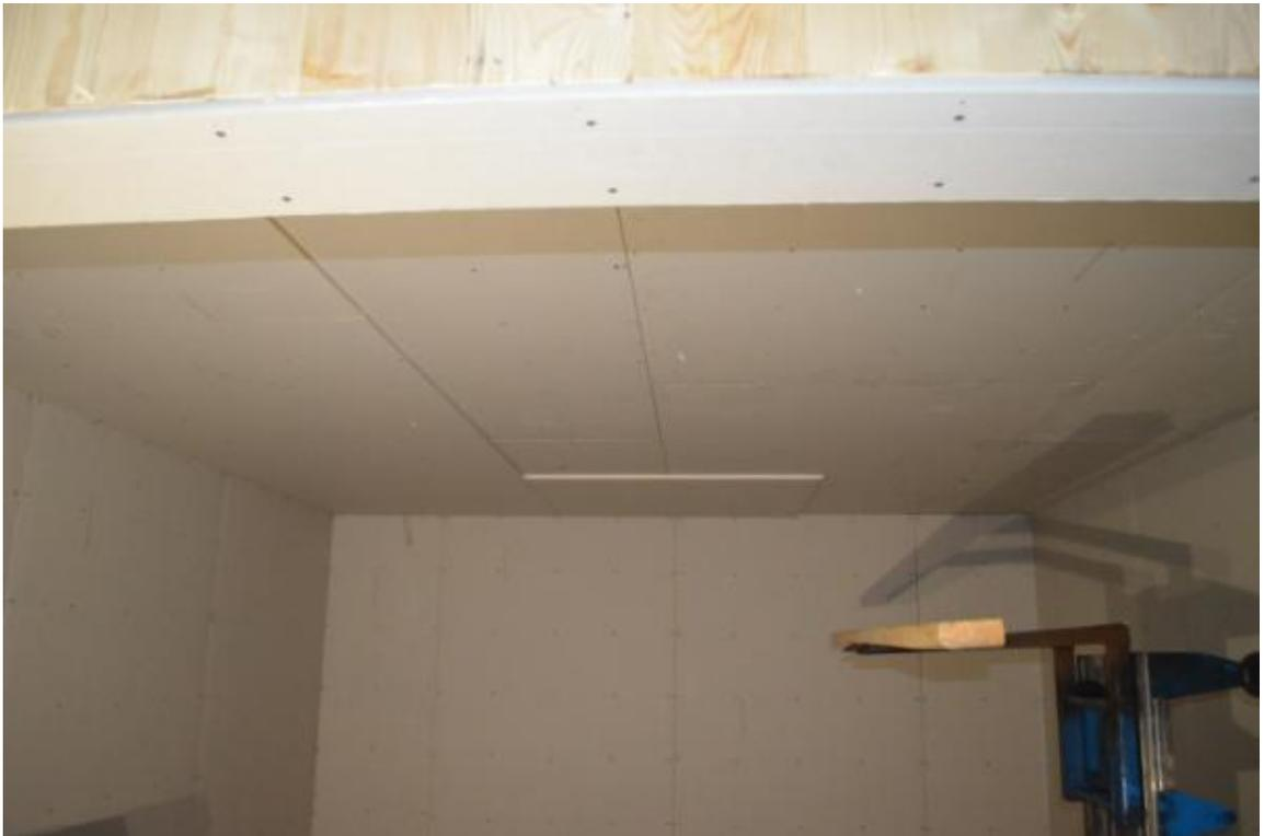
**Figure B-6. Face Layer of Gypsum Board on Ceiling.**
