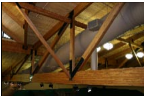
Figure 7 Glue-Laminated Timbers Used in Roof Truss
