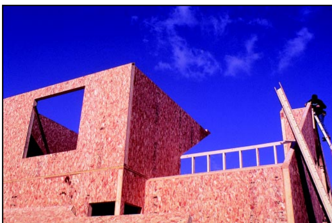
Figure 9 Wood Structural Insulated Panel (SIP) Installations
