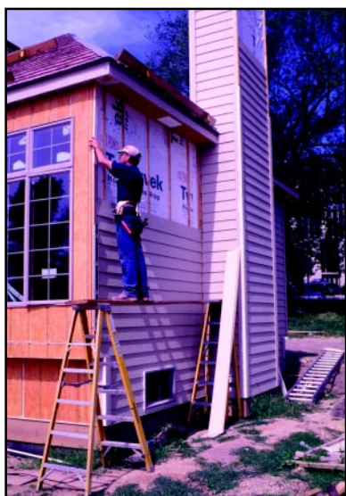
Figure 8b Siding Installation
