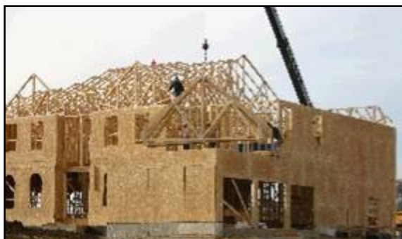
Figure 1 Roof Trusses
