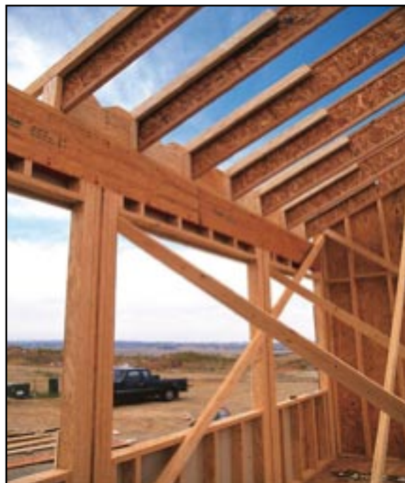
Figure 9 SCL Used as Header and Blocking
