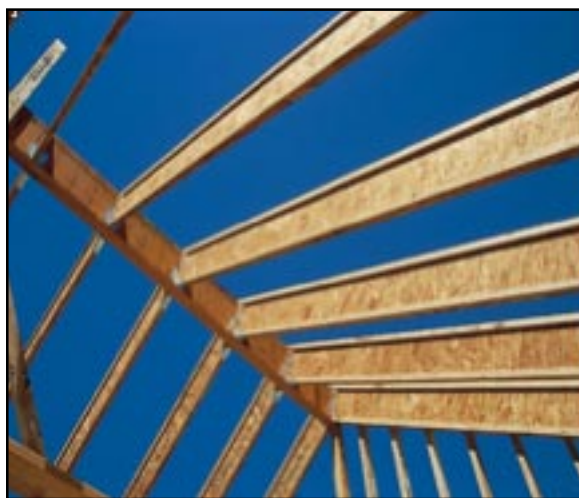
Figure 8 SCL Used as Ridge Beam in Roof
