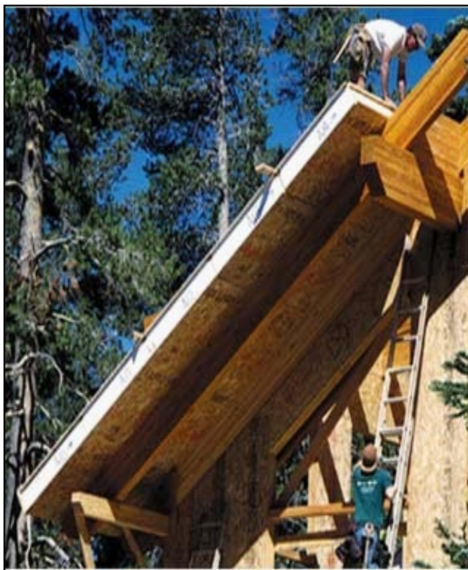
Figure 4 Structural Insulated Panel Roof Assembly
