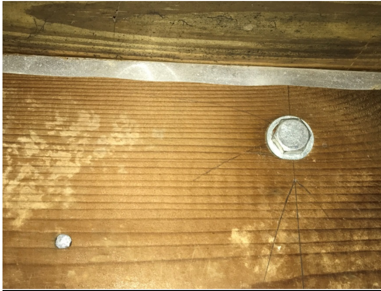
Figure 4. Section of a deck ledger with ½" diameter lag screw installed. (Photo by Frank Woeste)
