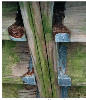
**Use the right joist hangers.** Although galvanized, the hangers on this seaside deck are rusty and nearing failure. Regular inspection of hardware is a good idea.
