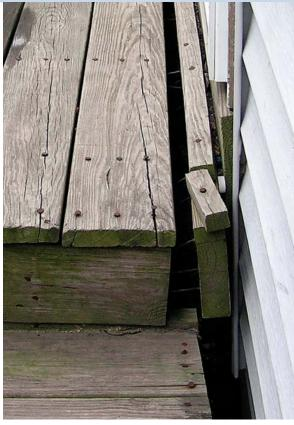
Nails alone don't do the job. This small deck was assembled by driving nails through the back of the ledger into the joists' end grain prior to installation. Toenailed joist-to-ledger connections are more common but also likely to fail
