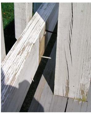
**Don't rely on nails.** This railing was just nailed to the outside of the posts. The nails eventually withdrew, and the railing pulled away.
