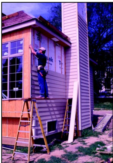
Figure 8b Siding Installation
