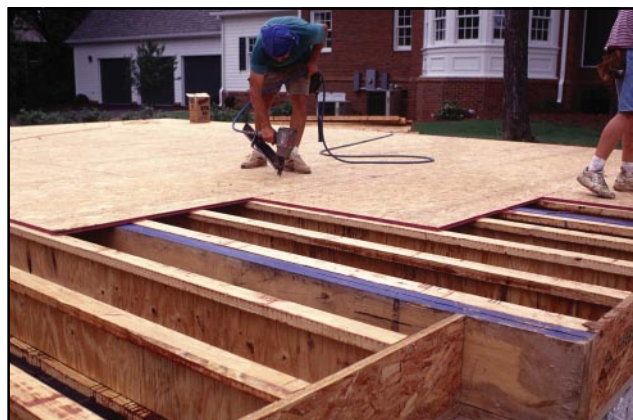
Figure 7 Single-Layer Floor Panel Installation
