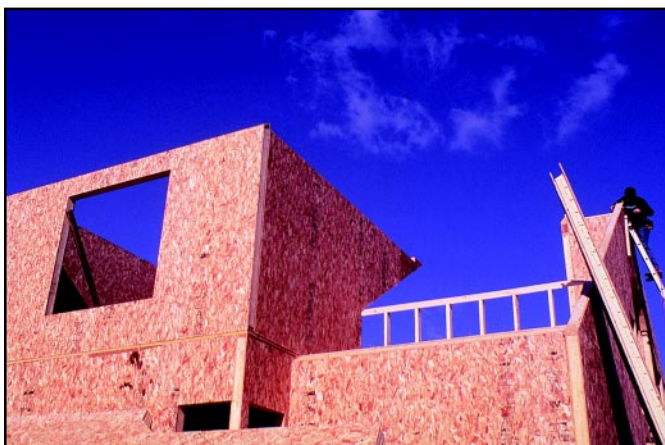
Figure 9 Wood Structural Insulated Panel (SIP) Installations
