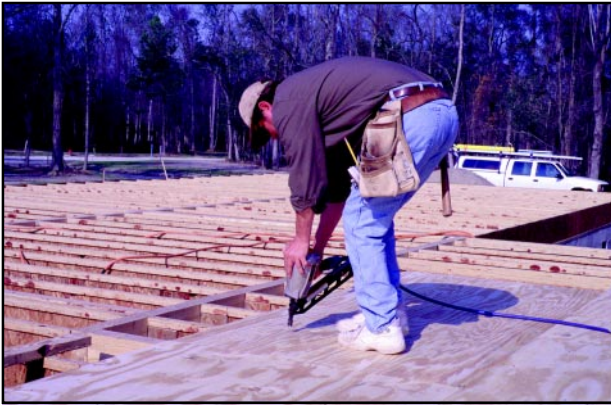
Figure 10b Floor Construction
