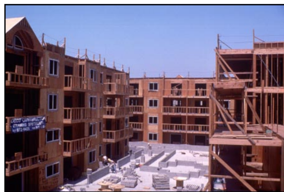
Figure 2 Wood-Framed Apartments under Construction
