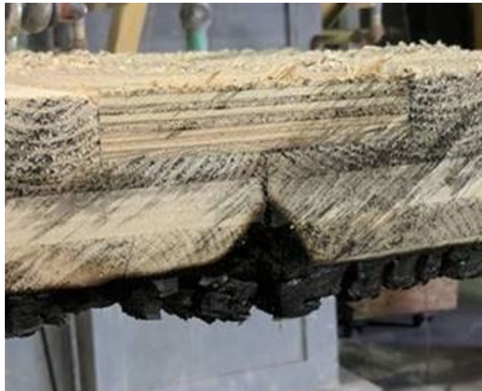
Figure 1-6. Example of char penetration at abutting edges of CLT floor panels (photo courtesy of Katerra).
