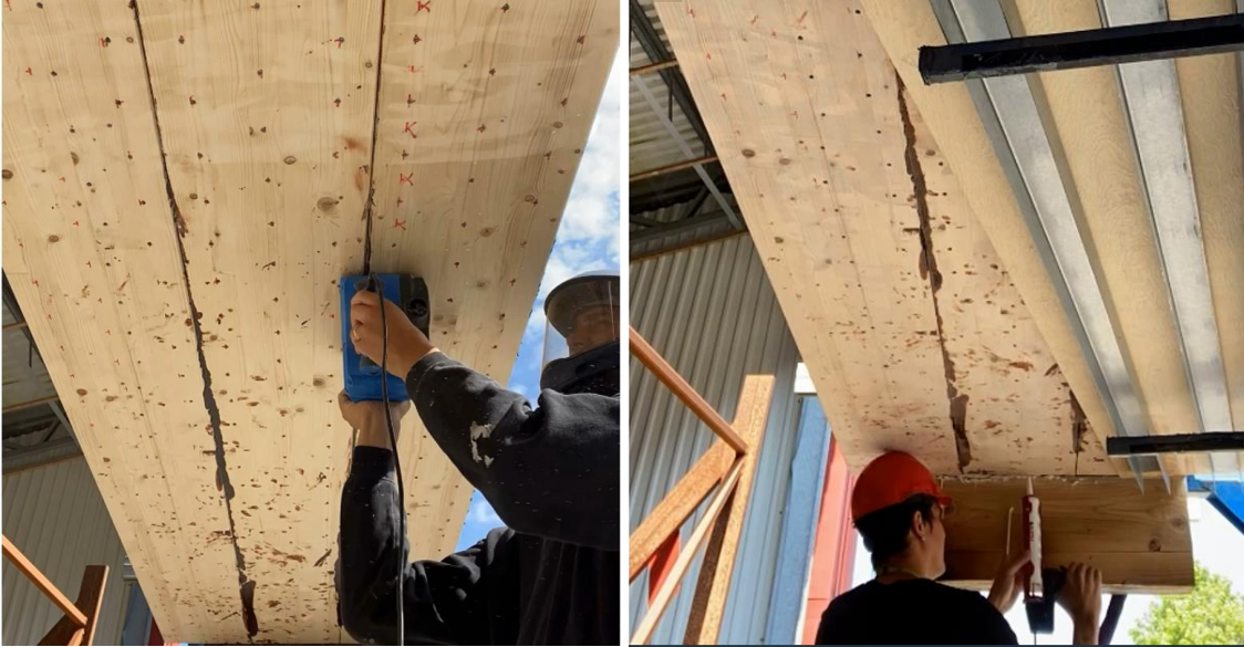
Figure 19: Sanding (left) and fire sealing the ceiling-wall joint (right)
