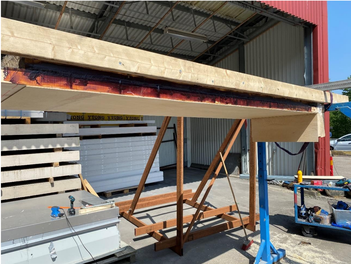
Figure 22: Specimen after rehabilitation work
