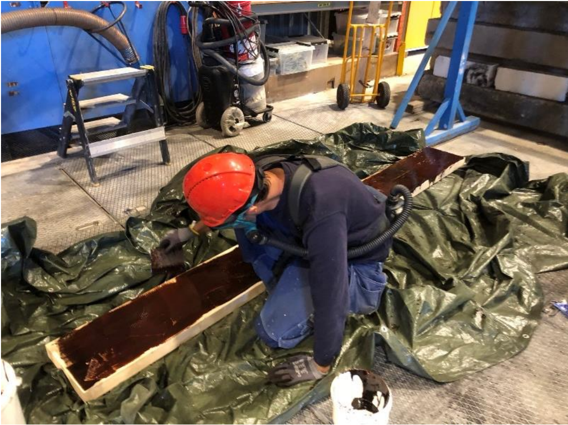
Figure 16: Applying adhesive on the lamella with a glue comb
