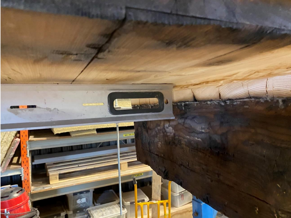
Figure 11: Checking the planeness of the surface at the corner
