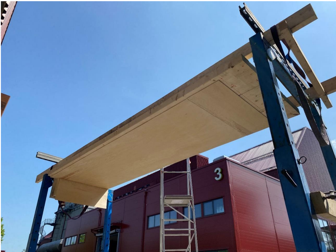
Figure 21: Specimen after rehabilitation work
