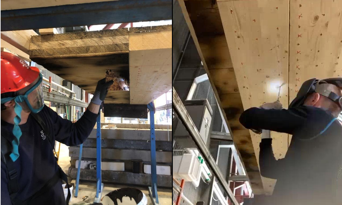
Figure 18: Scraping off pressed out glue (left) screw pressing (right)
