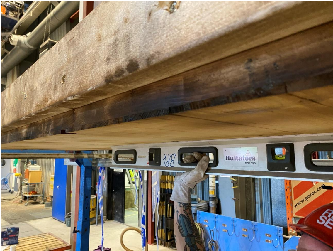
Figure 10: Checking the planeness of the surfaces
