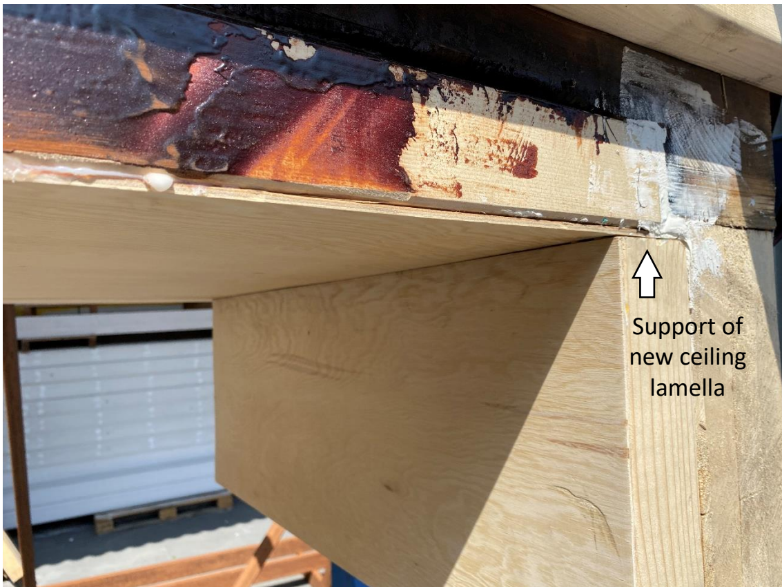
Figure 23: Ceiling-wall joint after rehabilitation work
