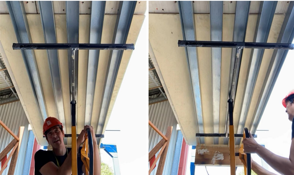
Figure 20: Putting a small amount of pressure with a panel lift and moving the lift's position a few times with 5 minute time intervals to compress at different locations.
