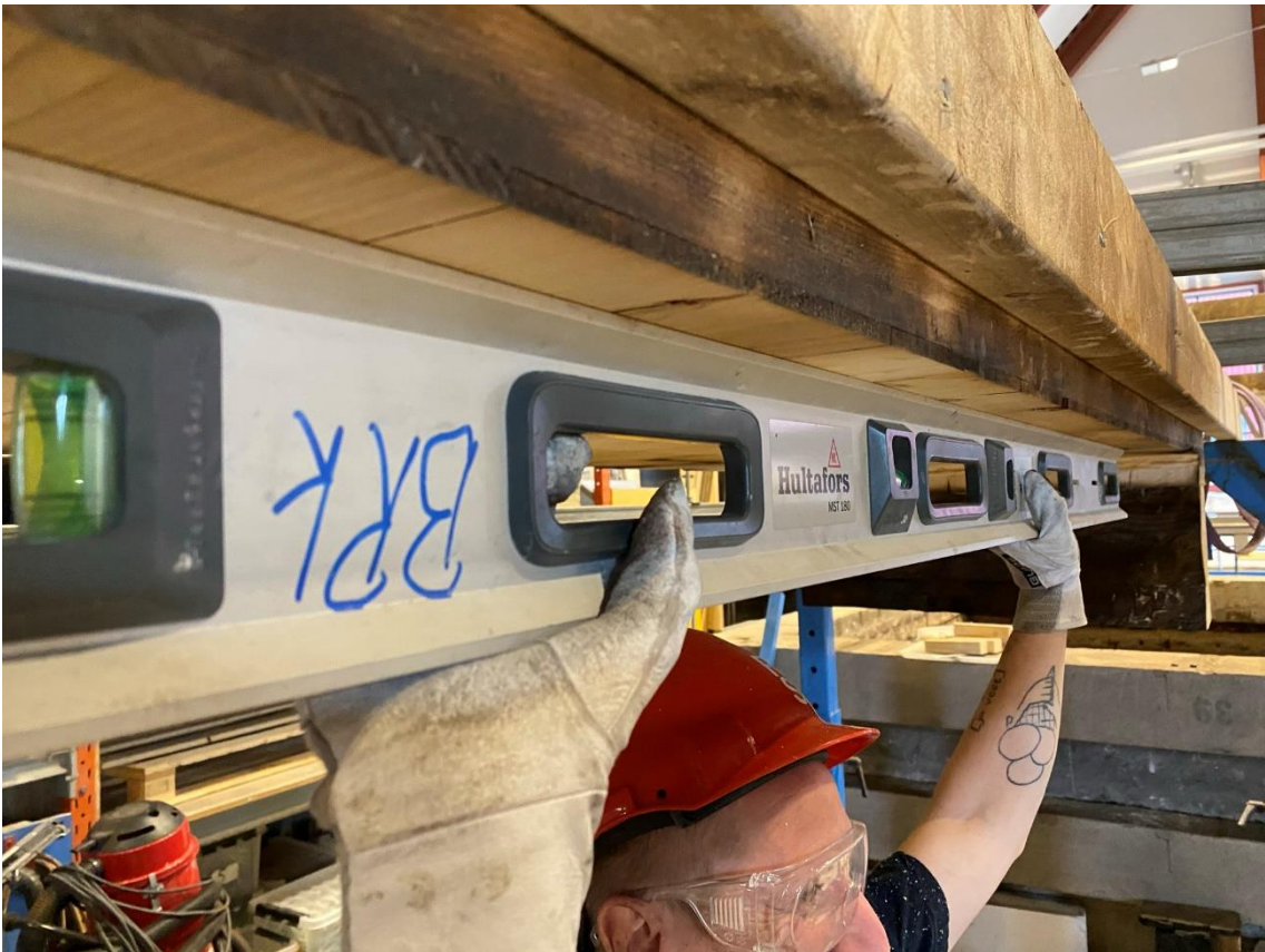
Figure 12: Checking the planeness of the surface
