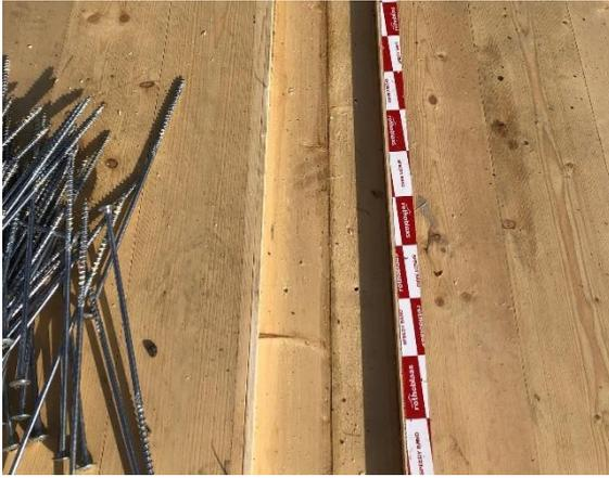
Figure 32: Photo after removal of spline board. Sealing method: 2x construction tape on top of spline boards (Test 1)
