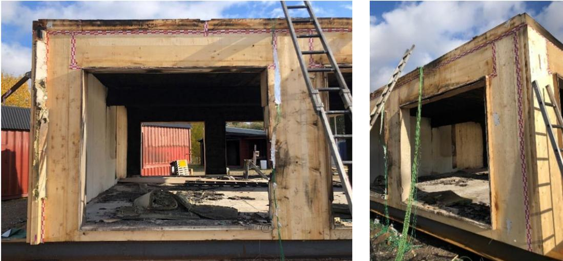
Figure F. 14. Test 4 – Left façade after removal of gypsum boards.
