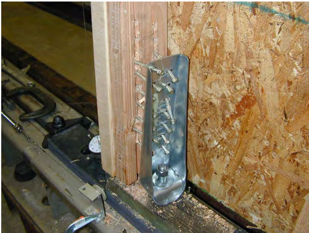
Figure 13. End stud failure at hold-down (Specimen B1)
