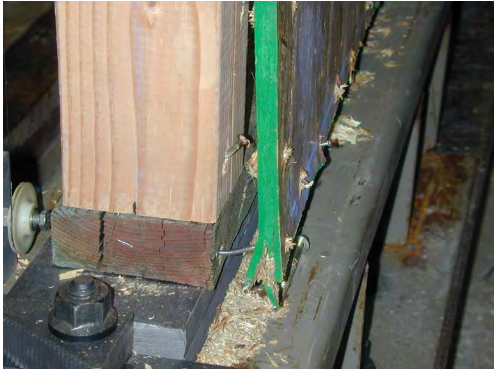
Figure 14. Failure showing split at end of sole plate (Specimen B1)
