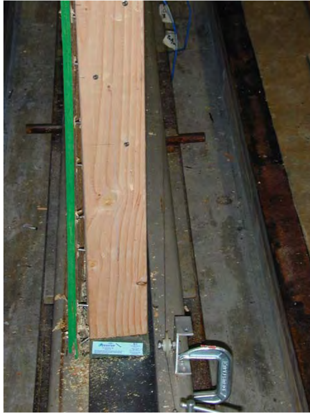
Figure 30. Sheathing separation from framing (Specimen D2)
