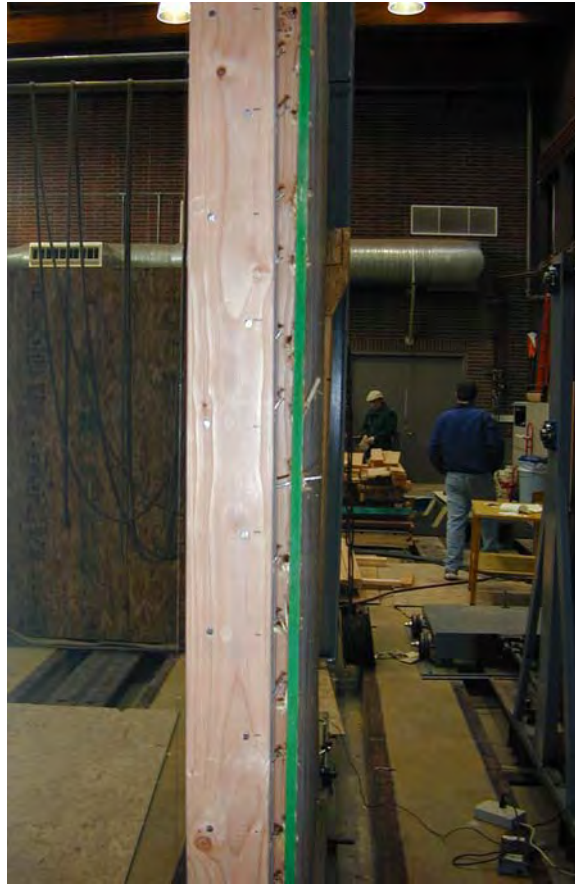
Figure 8. Sheathing edge pull-out (Specimen A2)
