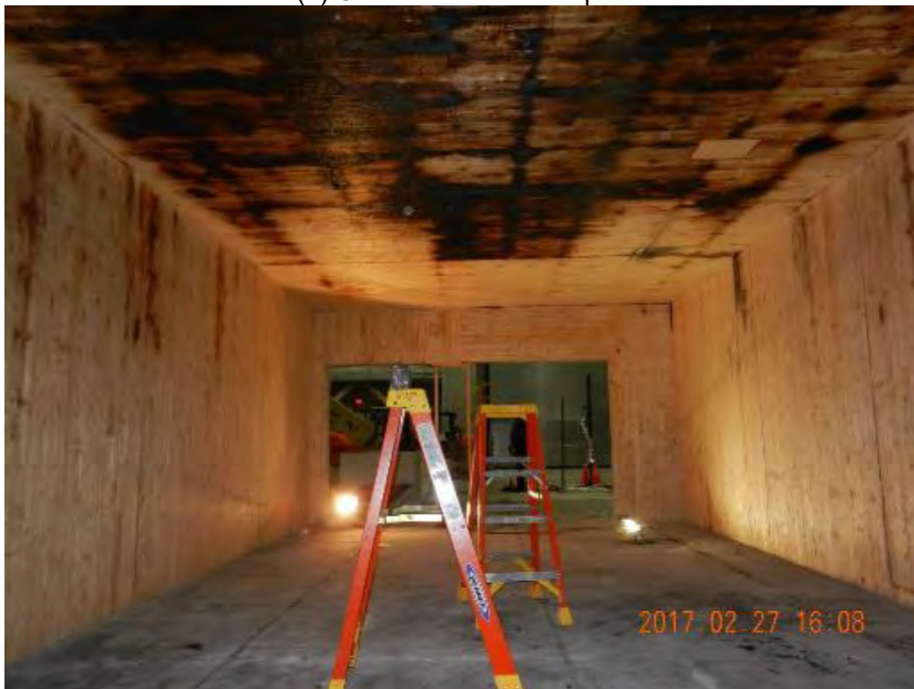
(b) CLT structure after repair
