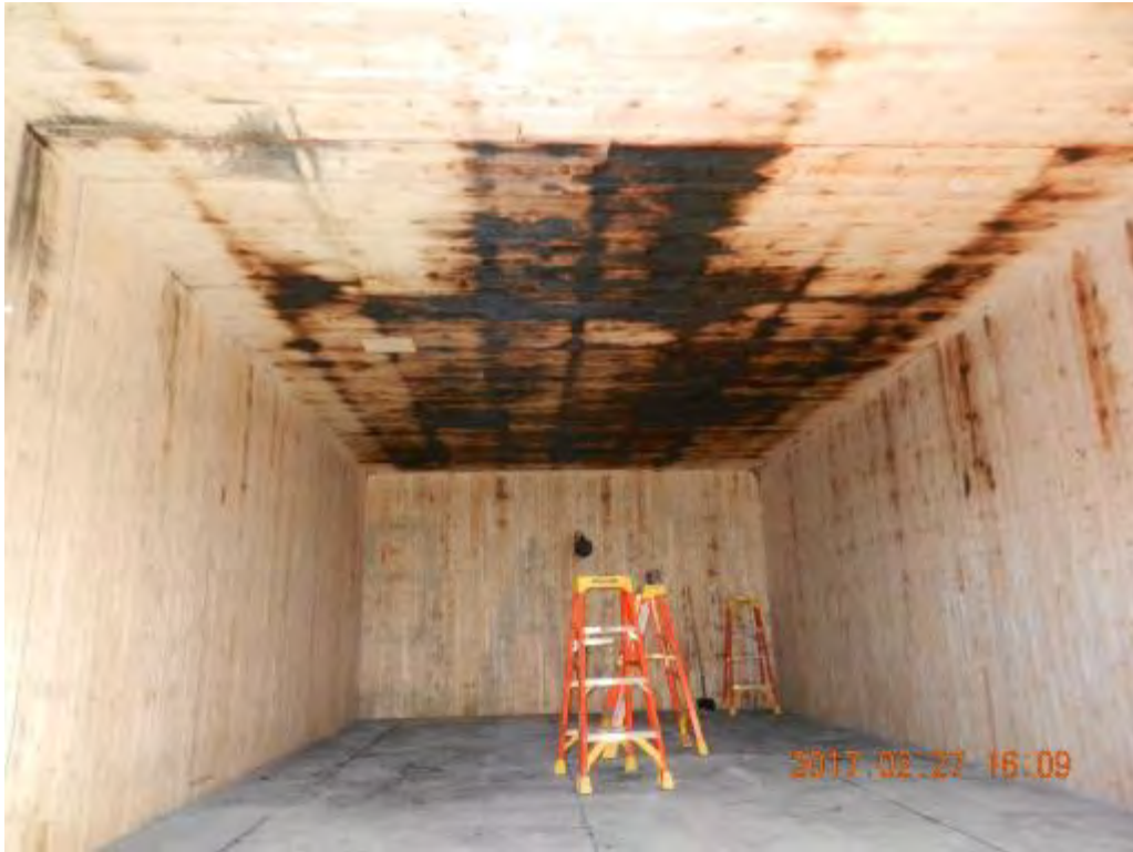
(a) CLT structure after repair
