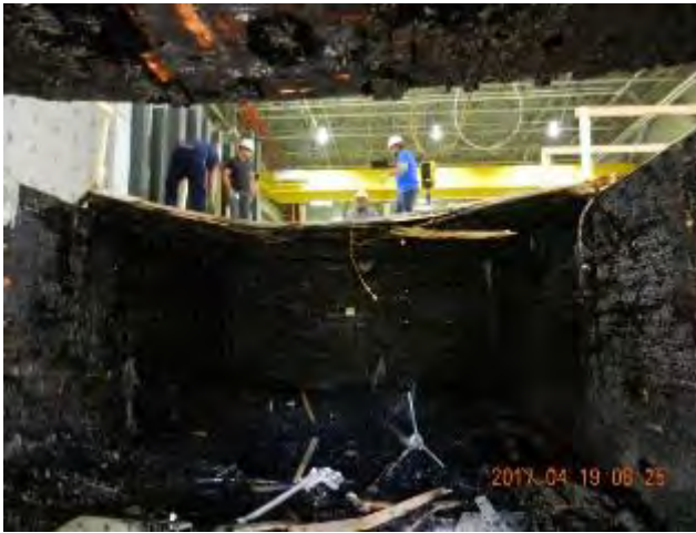
(a) Compartment interior surface
