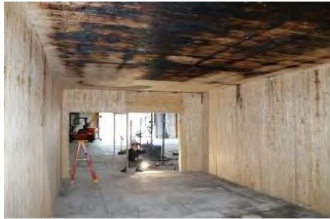
(b) after cleanup and removal of gypsum board
