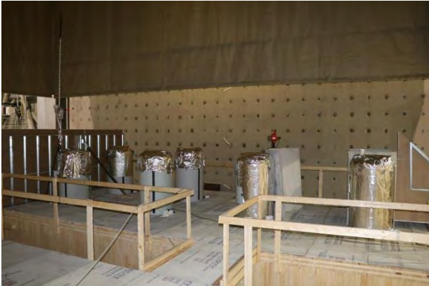
(a) cement board on top of ceiling
