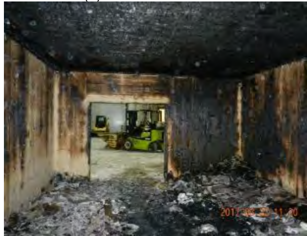
(d) interior with gypsum board removed
