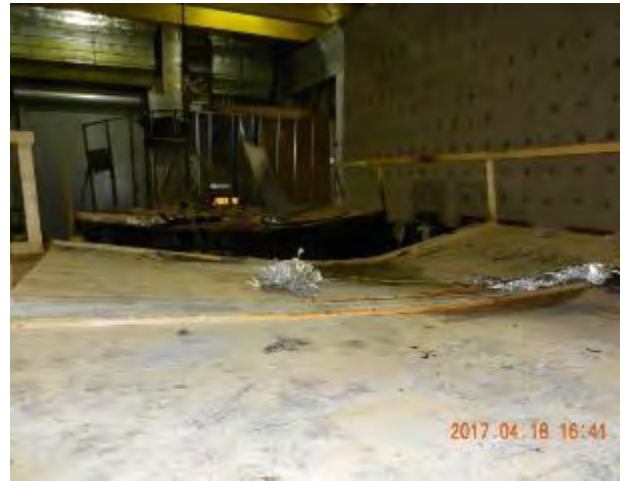
(b) Ceiling exterior surface
