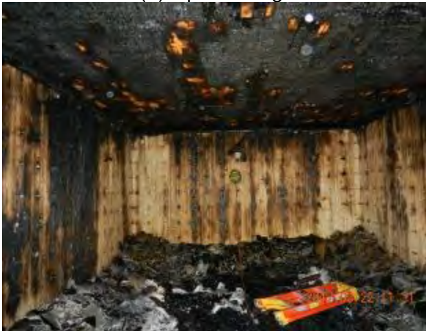
(c) interior with gypsum board removed
