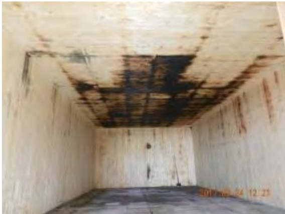
(a) after cleanup and removal of gypsum board
