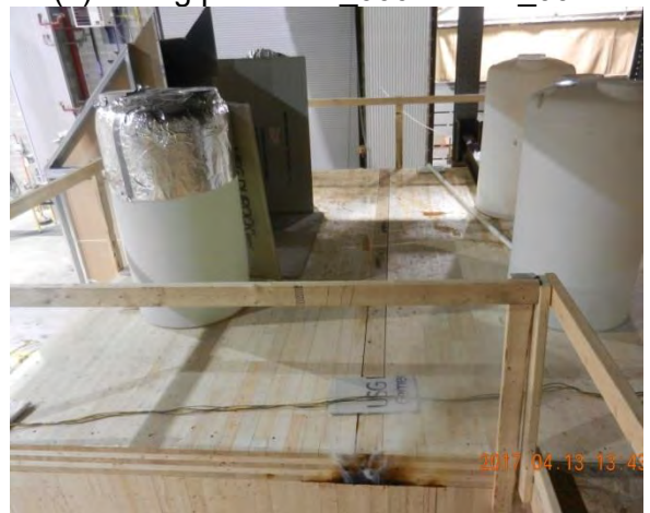
(f) ceiling panels 11_005 and 11_006
