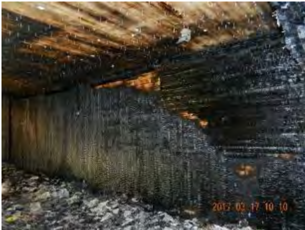
(c) W1 and ceiling after Test 1-3.
