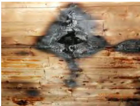
(c) joint of ceiling panels 11_006 and 11_007
