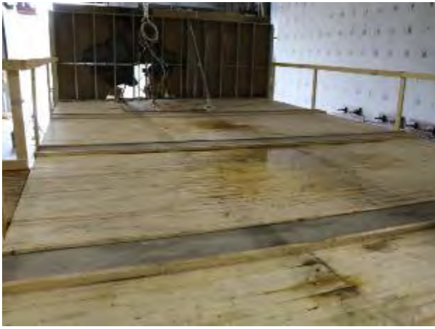
(a) top of ceiling
