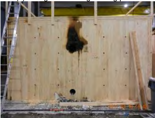
(e) drilled holes through wall panels
