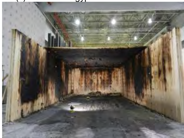
(e) during demolition
