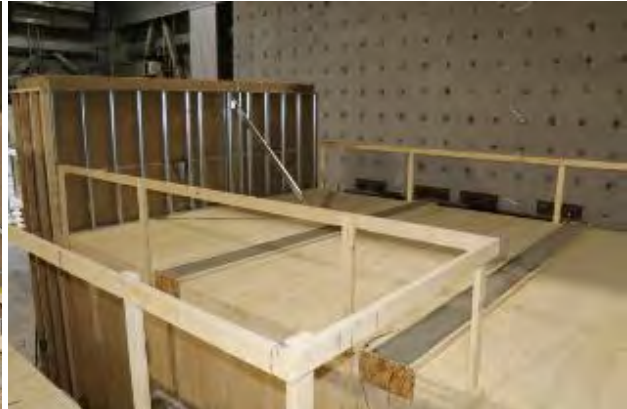
(b) gypsum concrete on top of ceiling joints
