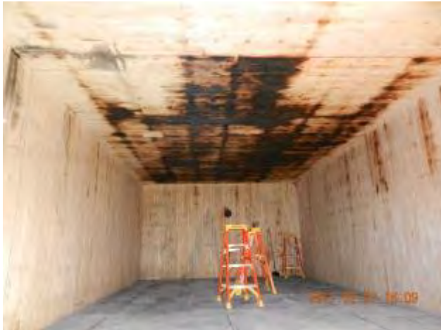
(a) W3, W4 W1 and ceiling CLT before Test 1-3.
