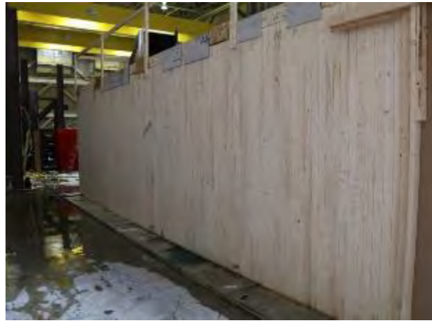
(b) exterior of W1 wall
