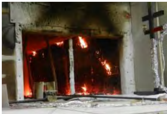
(g) exposed W1 at 240 min after 2 nd ply falling off
