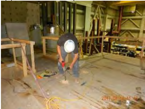
(c) drilling holes through ceiling panels
