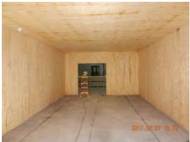
(h) after cleanup and removal of gypsum board
