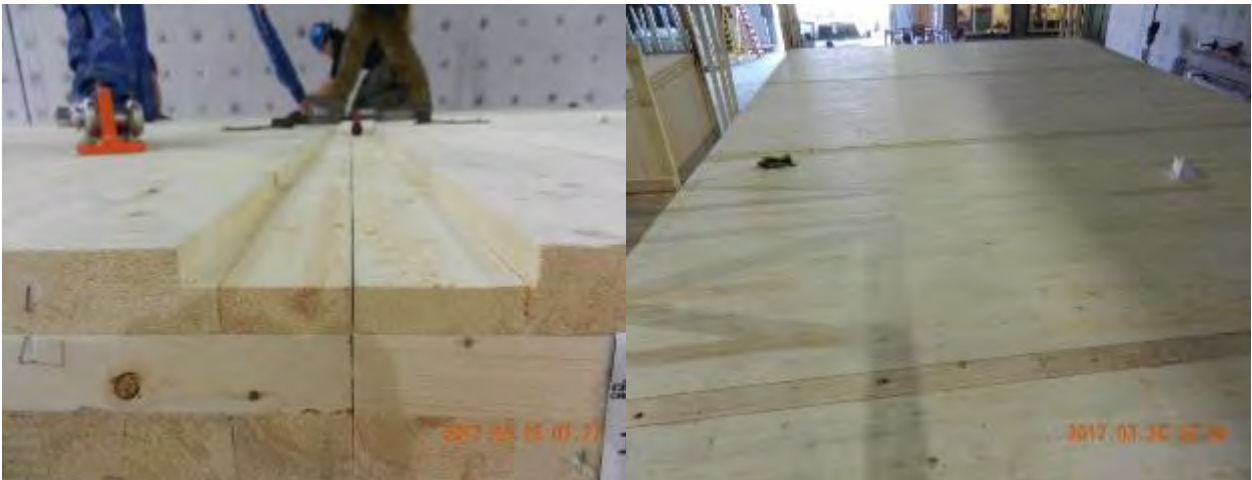
Figure 7. Ceiling panels connected with spline joints.
