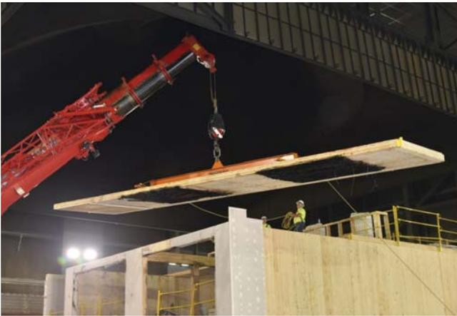
Figure 60. Second-level ceiling panel being removed after Test 2.
