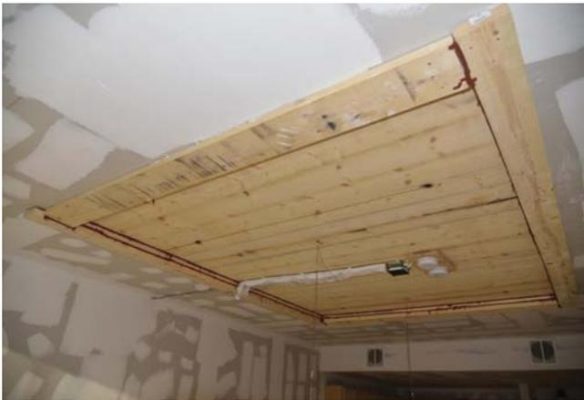
**Figure 33. Exposed cross-laminated timber ceiling in the living room for Test 2.**
