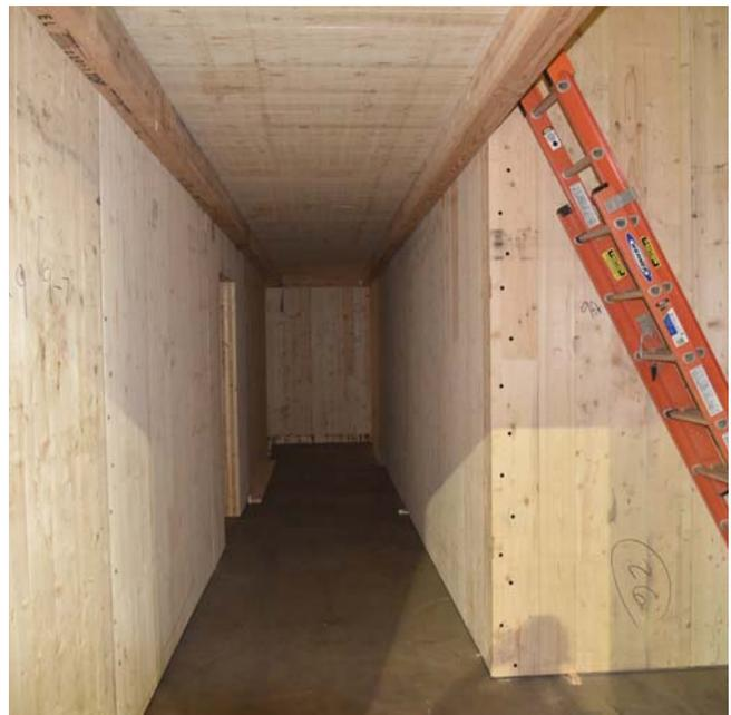
Figure 12. Ledgers in the corridor along Walls C and F.
