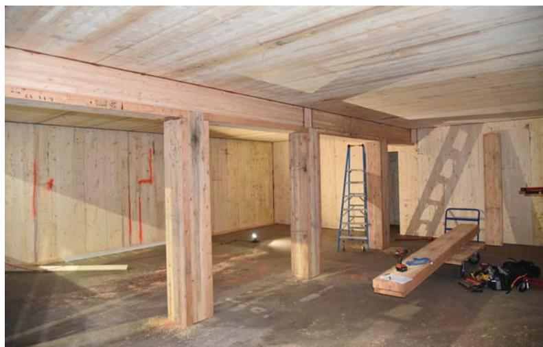
Figure 16. Wood-protected support columns and beams on first floor.
