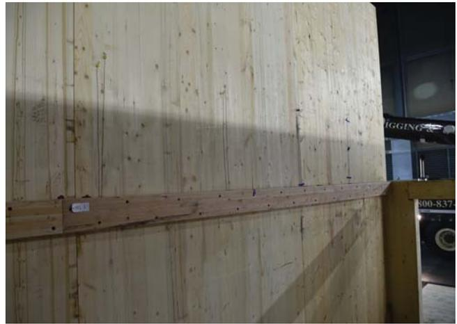
Figure 10. Ledger on Wall D to support second-level floor in the apartment.
