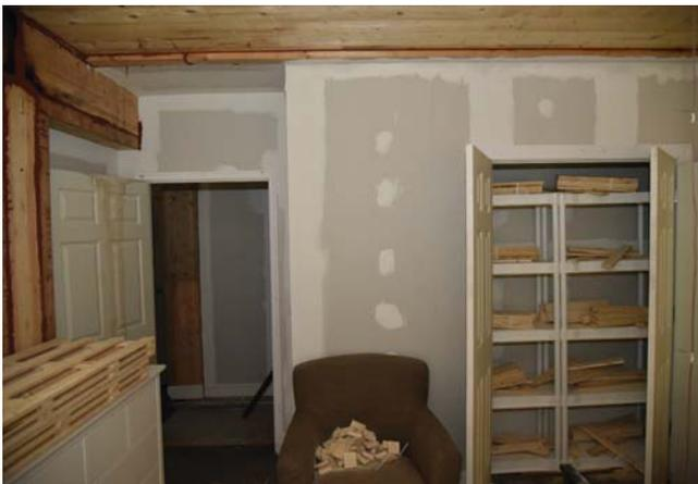
Figure 39. Wood trim placed along the edge of the gypsum wallboard on the ceiling.
