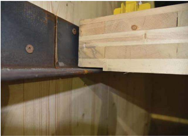
Figure 8. Cross-laminated timber floor panel on steel angle.
