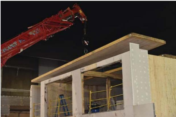
**Figure 17. A second-level ceiling panel being installed.**
