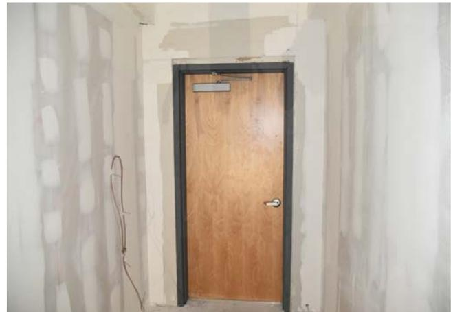
Figure 24. Fire door assembly between corridor and stairwell.
