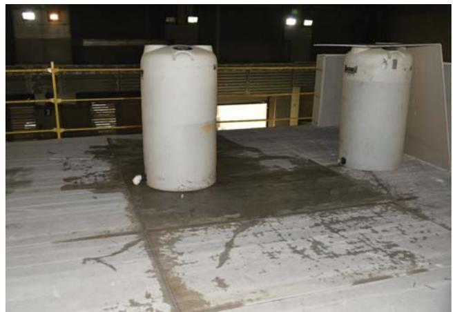
Figure 55. Water tank that leaked.
