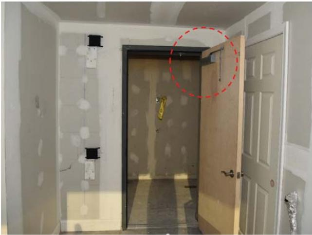
Figure 98. Automatic door closer not attached for Test 3.
