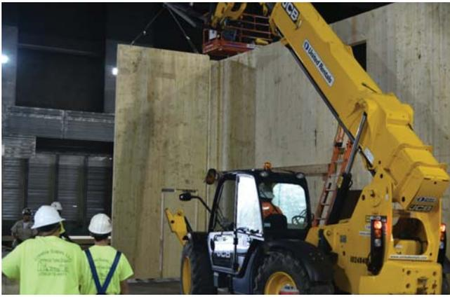
Figure 4. Installation of a cross-laminated timber wall panel.
