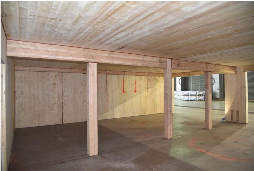
Figure 13. Original midspan beams and support columns on the first floor.
