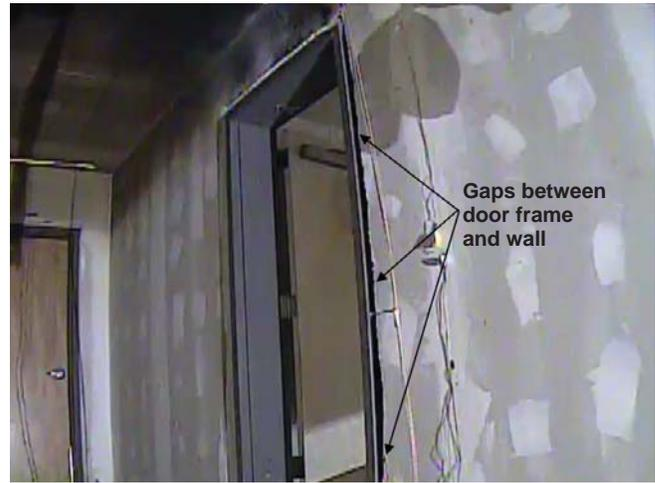
Figure 99. Gaps between door frame and wall.
