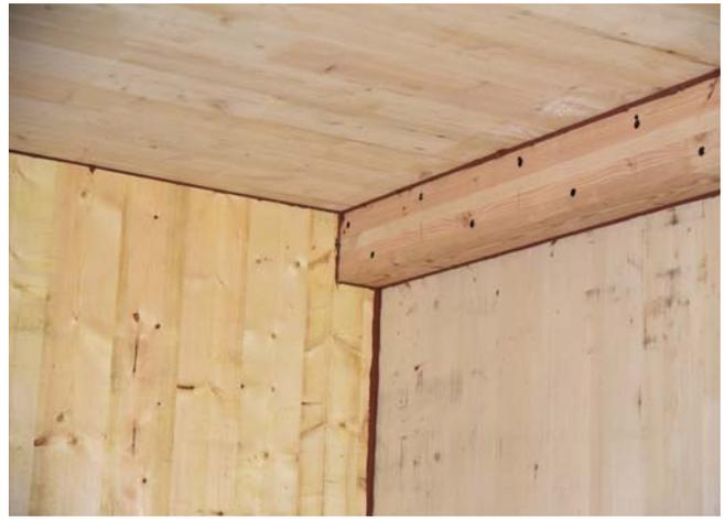
Figure 40. Cross-laminated timber joints sealed with intumescent firestop sealant.
