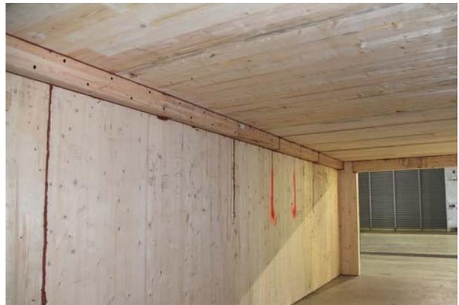
Figure 11. Second-level floor on top of the ledger.
