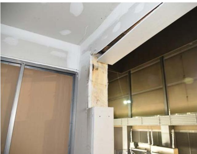
Figure 62. Section of damaged cross-laminated timber removed from Wall A on second floor.
