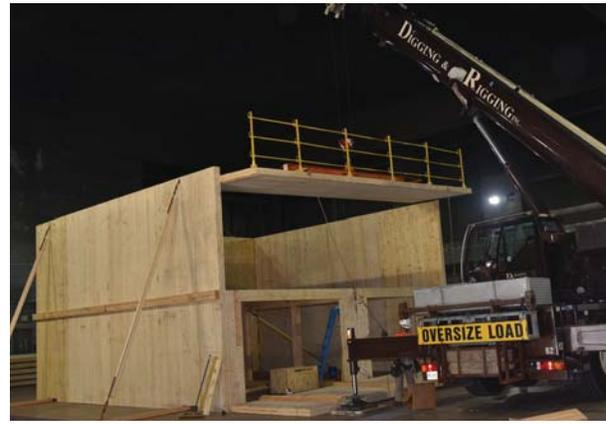
Figure 6. Installation of a second-level floor panel.
