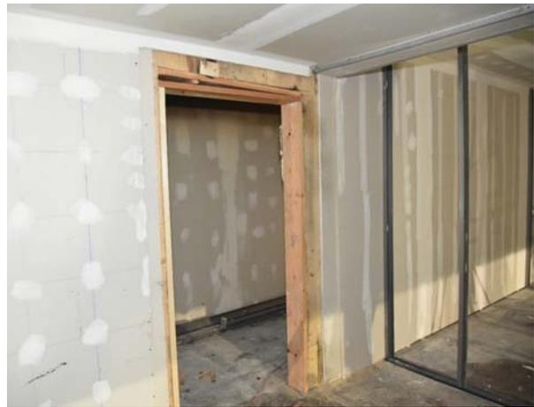
Figure 64. Repair to damaged area around second-level apartment door.
