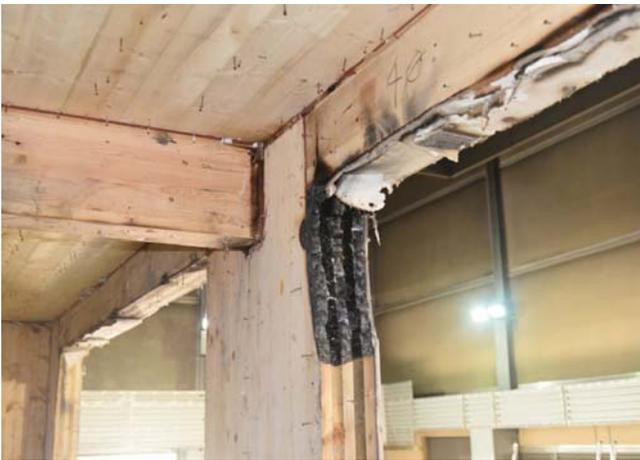
Figure 61. Localized section loss caused by charring on Wall A at the living room opening on the second floor.
