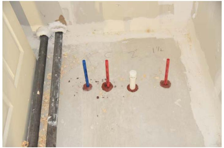
Figure 31. Plumbing penetrations in the utility room on second-floor level.
