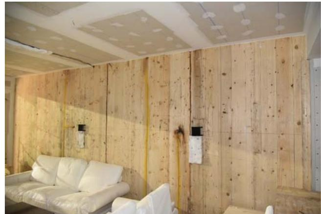
**Figure 35. Exposed cross-laminated timber wall in the living room for Test 3.**
