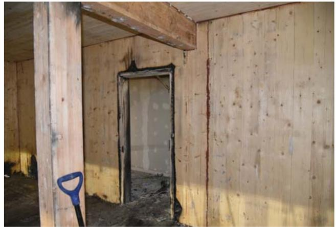
Figure 63. Localized section loss caused by charring around apartment door frame on the second floor.
