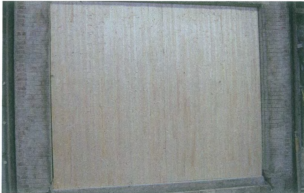
Exposed Side – CLT Wall Construction
