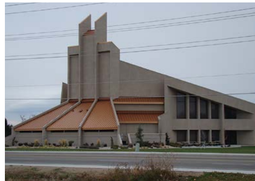
Figure 14—Type III construction
