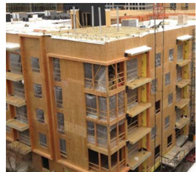
Figure 34—Wood exterior balcony
