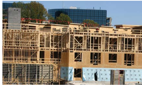
Figure 10—Type V construction
