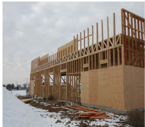
Figure 43—Wall bracing
