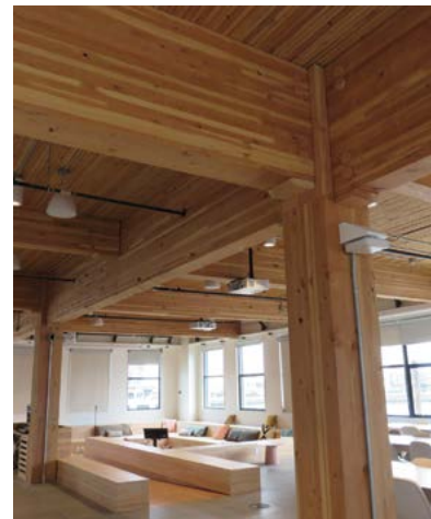
Figure 38—Beam column connection
