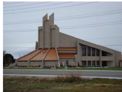
Figure 11: Type III Construction
