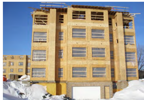
Figure 9: Type V Construction
