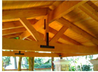
Figure 10: Type IV Construction
