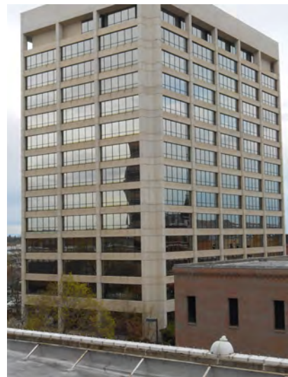
Figure 12: Type I Construction
