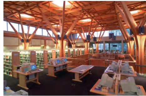
Figure 10: Type IV Construction
