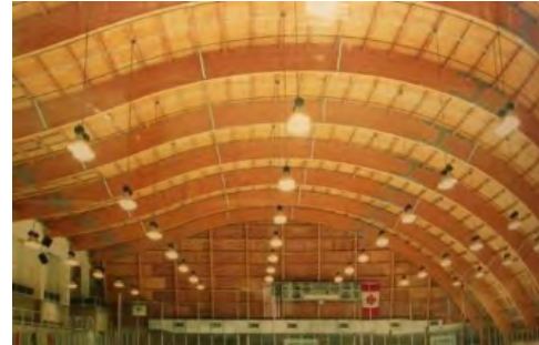
Figure 16: Heavy Timber Construction
