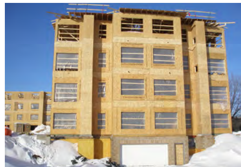
Figure 9: Type V Construction
