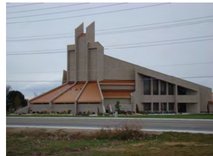
Figure 11: Type III Construction
