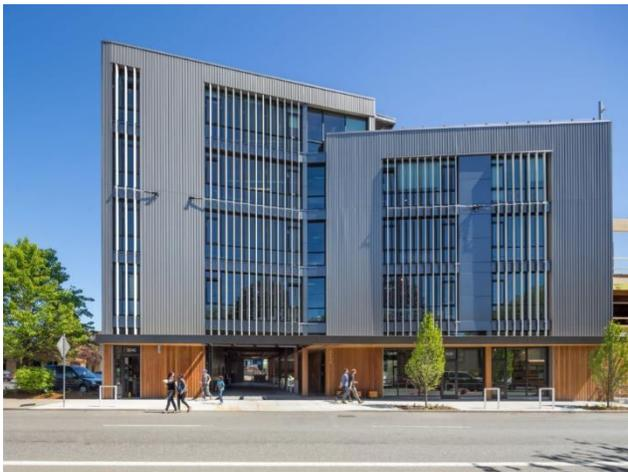
The Radiator is one-third of the Portland, Oregon, office park known as One North. It was designed by Path Architecture, along with general contractor (and developer) Kaiser Group, Munzig Structural Engineering, and PAE Consulting Engineers (for mechanical work). Glued-laminated timber (glulam) was an important part of its design, both from functional and aesthetic perspectives.
