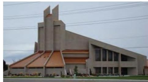
Figure 5: Type III Construction
