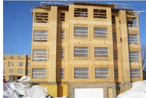
Figure 3: Type V Construction
