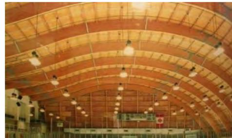
Figure 10: Heavy Timber Construction
