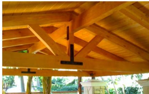
Figure 3: Type IV Construction
