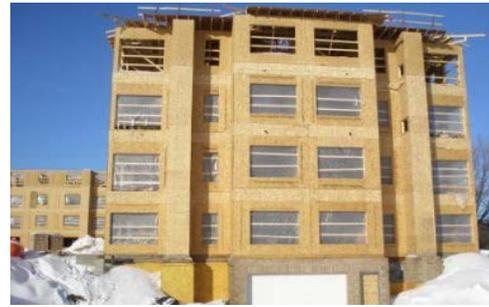
Figure 2: Type V Construction
