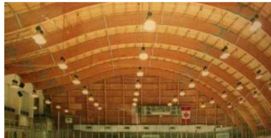
Figure 13: Heavy Timber Construction
