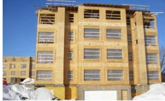
Figure 2: Type V Construction
