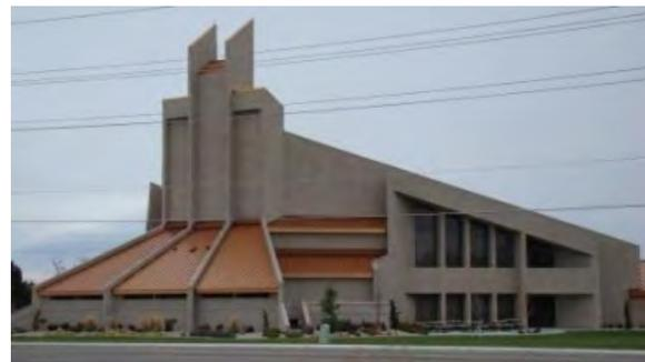
Figure 4: Type III Construction
