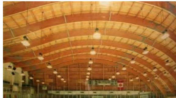
Figure 9: Heavy Timber Construction
