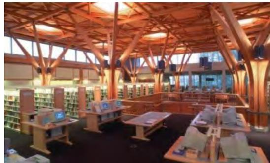
Figure 3: Type IV Construction
